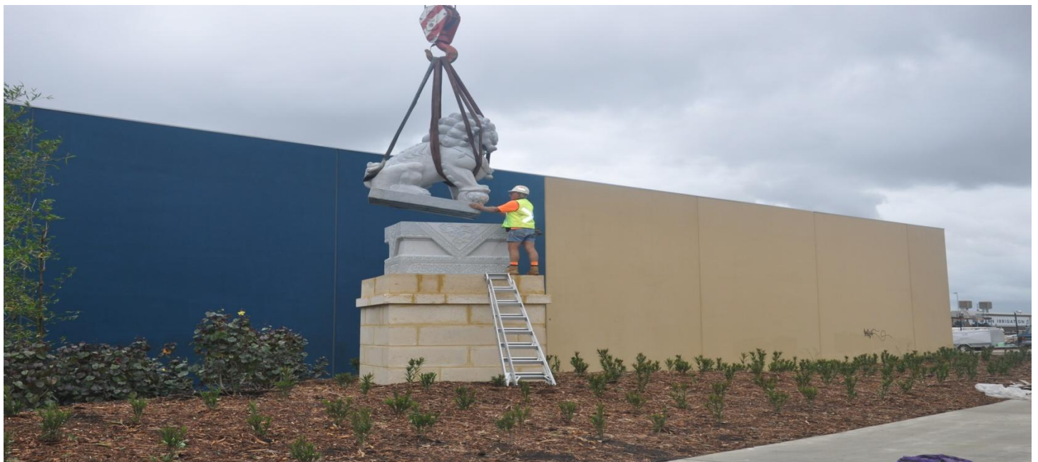
One of the traditional lions being installed on Friendship Way
