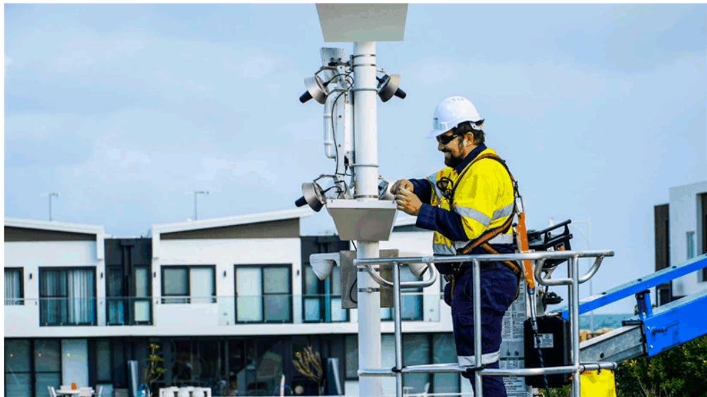
Image 5: LED streetlight upgrade, Port Coogee, June 2020
