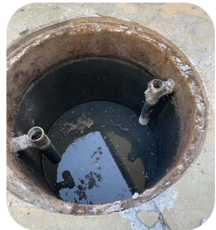
Septic Tank to decommission.
