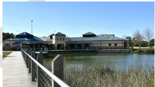
Figure 35. Beeliar Community Centre
