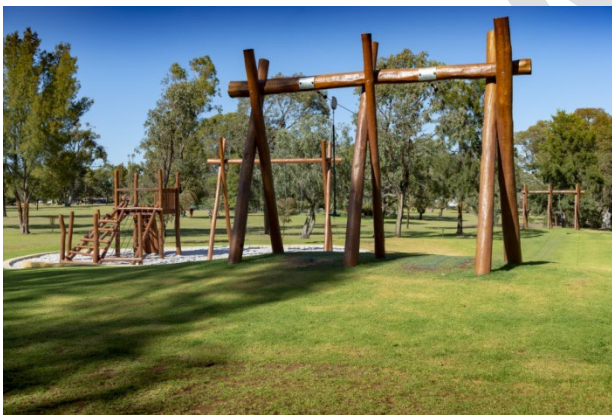
Figure 32. Improvements to MacFaul Park, Spearwood identified in the Phoenix Revitalisation Strategy and implemented
