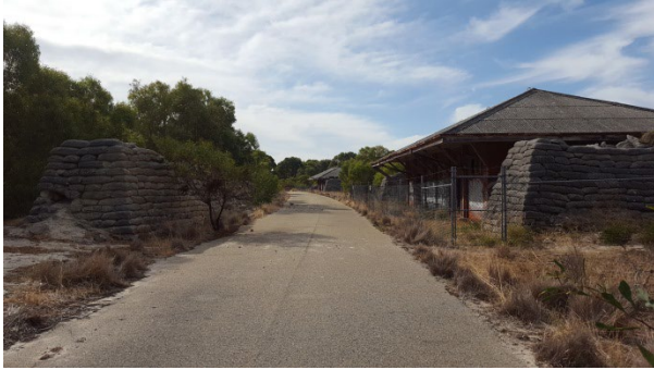
Figure 26. Remaining munition magazines, Woodman Point
