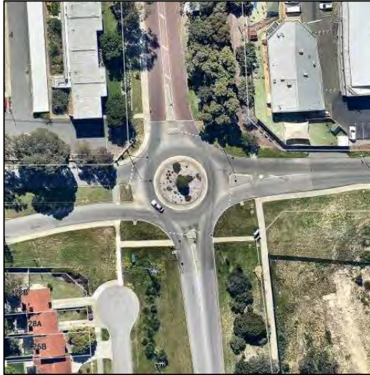
Figure 7.5: Existing Coolbellup Avenue / Cordelia Avenue Intersection (Source: Nearmap)
