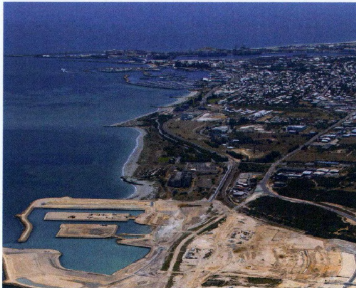
Figure 07_Aerial of the Cockburn Coast Development Area looking North
