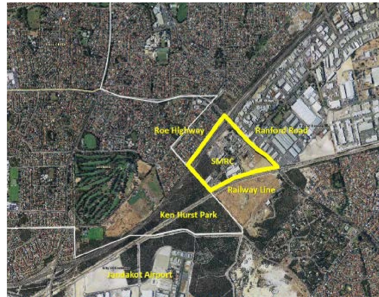
Recommended boundary adjustment for the parcel of land containing the SMRC's RRRC for inclusion into the City of Melville
