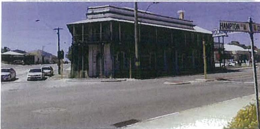
Figure 2: Subject site looking south east from Cockburn Road
