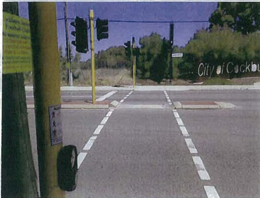
Figure 21: Pedestrian crossing facility at the signalised intersection of Rockingham Road/ Cockburn Road
