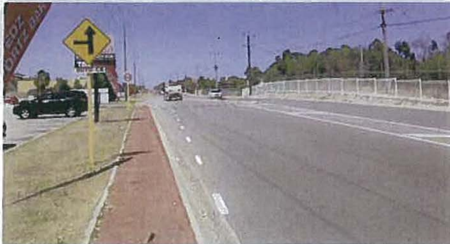
Figure 18: Speed limit of 60 Km/hr along Cockburn Road
