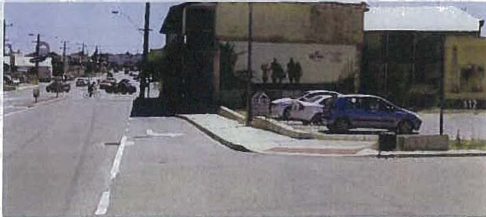
Figure 7: Existing Cockburn Road crossover showing the short left turn slip lane facility
