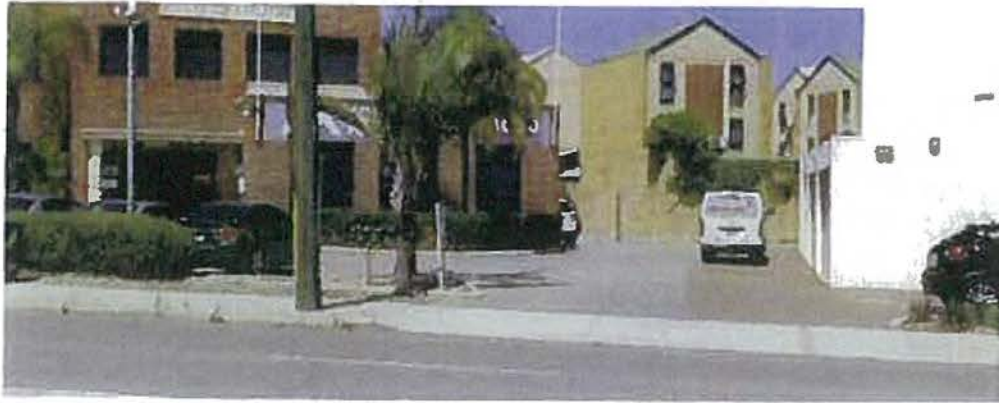
Figure 8: Existing Rockingham Road crossover
