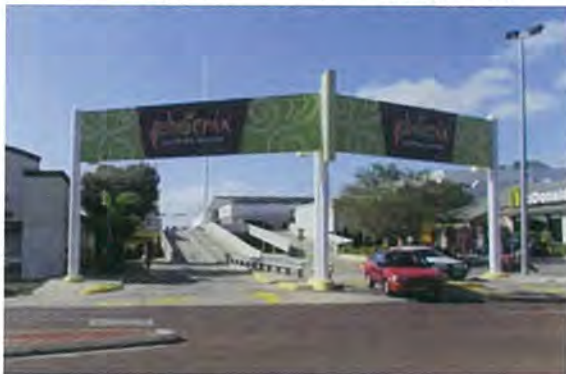
Figure 17. Rockingham Road vehicle entrance to upper deck parking - relies on signage
