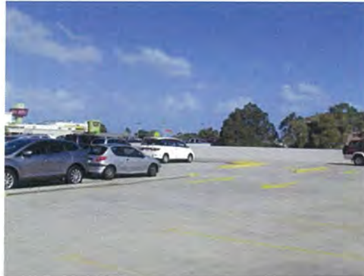
Figure 38. Existing expansive upper deck car parking
