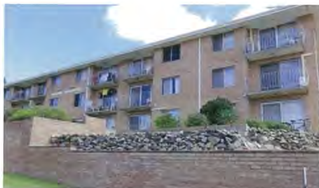
Figure 23. Glendower Way, Spearwood – 24 single bedroom apartments
