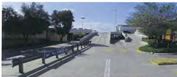
Figure 16. Ramp from Rockingham Road
