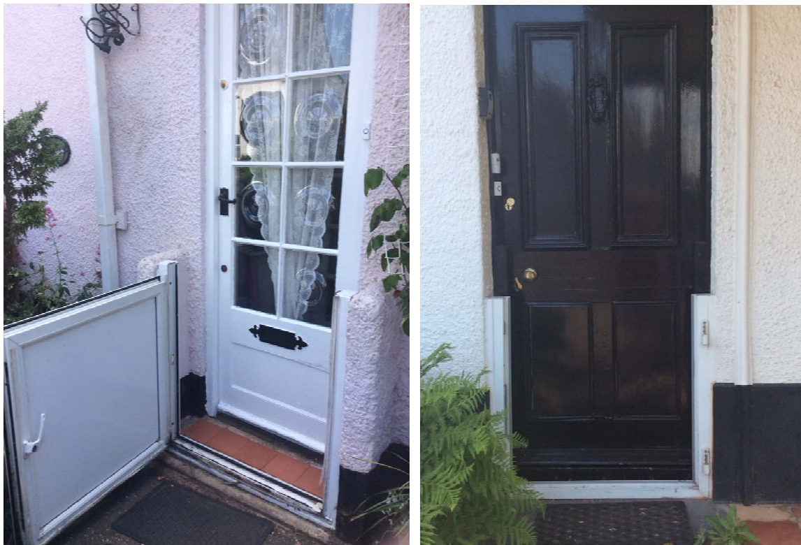
Flood gates on heritage properties are a common inundation accommodation treatment in the United Kingdom
