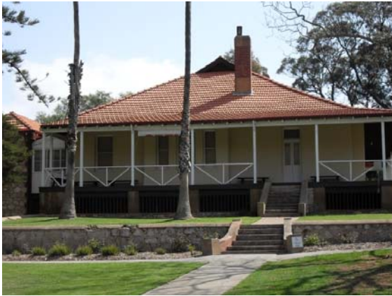
Figure 19 Azelia Ley Homestead Source: City of Cockburn Local Government Inventory
