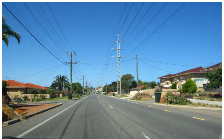
Figure 12: Existing high voltage power lines along Hamilton Road.
