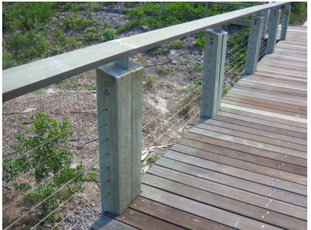
Figure 19: Boardwalk at Salt Estate, Kingscliffe, NSW
