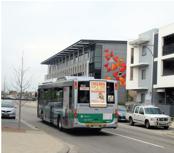
Above: The emerging Cockburn Central Regional Centre provides a mix of residential and commercial uses with good links to a range of transport options.
