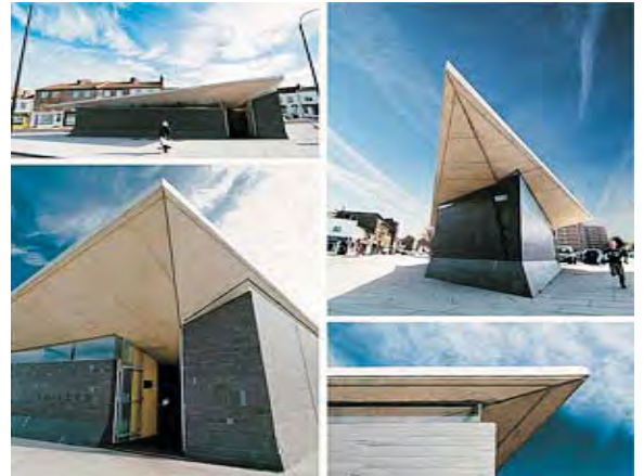
Example of Toilet Block designed as a feature within the site.
