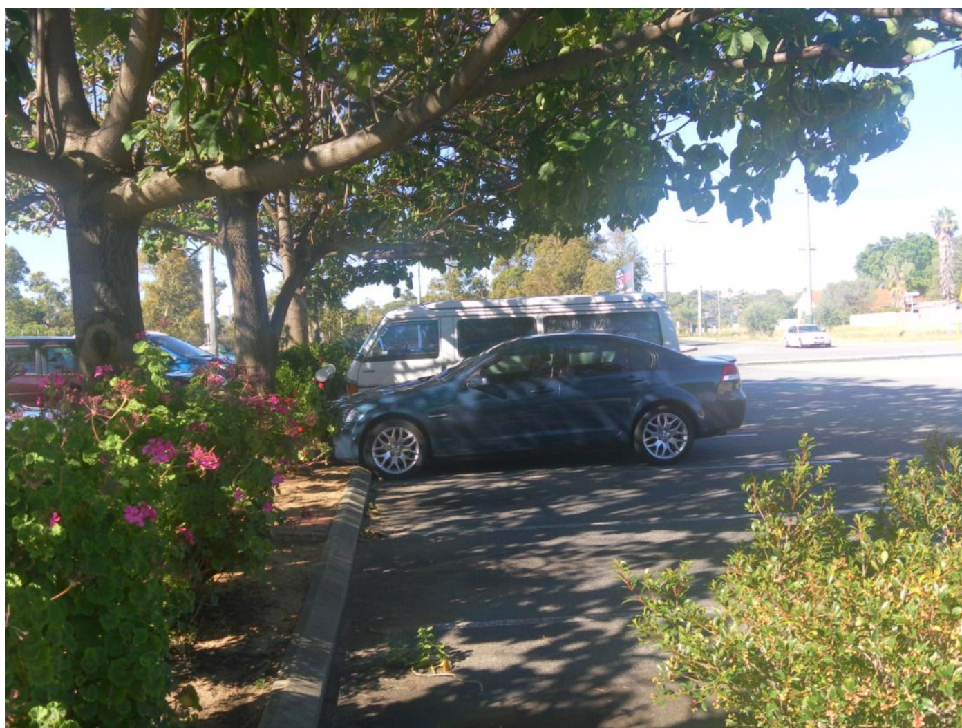
Photograph 8 and 9 (above and right) – Adoption of sound design practices creates shadier more sheltered environments using fewer resources. These car parks are cheaper to build and cheaper to maintain and create more shelter from the wind and sun. Note that in the IGA car park, Rockingham Road, Hamilton Hill (above) large trees are planted every three or four bays, much more than required by Town Planning Scheme 3.
