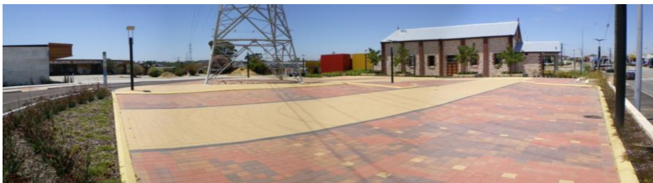
Photograph 3. Using the dimensions of the parking bay to determine paving block colours no painted line marking (a maintenance item) is required to organise car parking in this car park.
