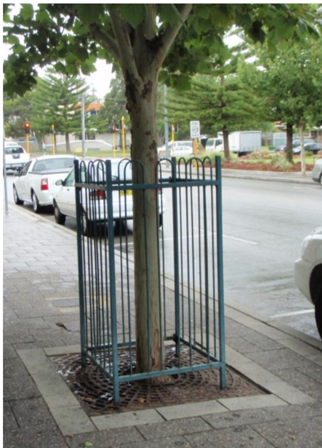
Photograph 10. Cast iron tree grates and steel guards protect the tree, provide a well for irrigation water to collect in, reduce the likelihood of the tree's roots damaging the paving, and prevent pedestrians tripping over the tree pit. The grate should be supported beneath with a steel frame, and the paving edges must be thickened or precast units must be haunched to provide a strong edge beam to the pit (example on right shows consequence of a failure to adequately haunch).
