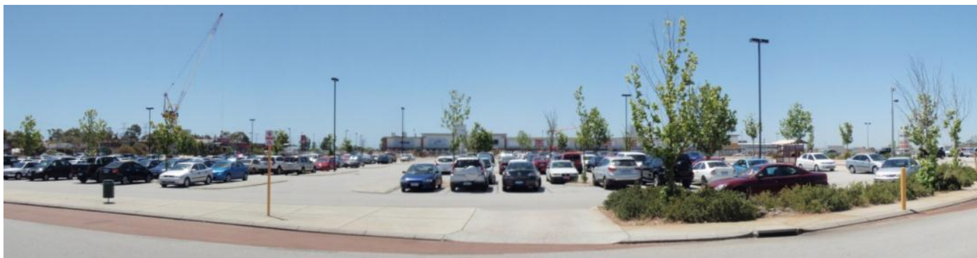
Photograph 6 and 7 (above 6 and right 7) - Poor exploitation of the potential offered to the designer by AS2890.1 often leads to expensive, wasteful design outcomes and low quality environments. 10 years after construction the trees in the Gateways Shopping Centre, Cockburn Central have not grown, many have died and large areas of asphalt are never driven on.
