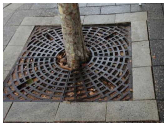
Photograph 10. Cast iron tree grates and steel guards protect the tree, provide a well for irrigation water to collect in, reduce the likelihood of the tree's roots damaging the paving, and prevent pedestrians tripping over the tree pit. The grate should be supported beneath with a steel frame, and the paving edges must be thickened or precast units must be haunched to provide a strong edge beam to the pit (example on right shows consequence of a failure to adequately haunch).
