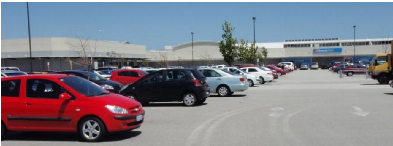
Photograph 5. This parking aisle at Gateways in Central Cockburn contains 39 bays. Chapter 2.3.3 Parking Aisle Length of AS2890.1 Off Street Parking facilities allows up to 40 spaces in an aisle. Aisles any longer than this encourage circulating traffic to idle in the aisles waiting for spaces to appear, rather than circulate from aisle to aisle. This makes the car park much less efficient and less attractive for visitors.
