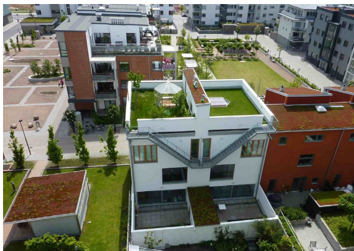
Example of screened building services for protection of amenity for communal open space
