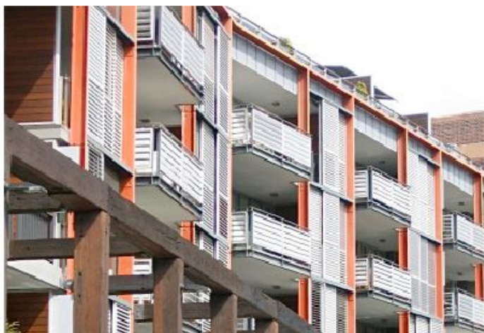
There is the potential for alternative methods to satisfy street character and front setbacks.
