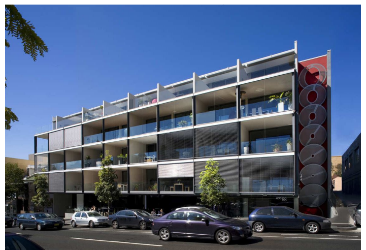
Example of shading devices promoting building character through articulation and material variety.
