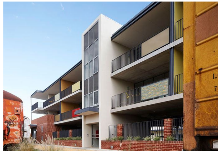
Example of a clearly defined pedestrian entry
