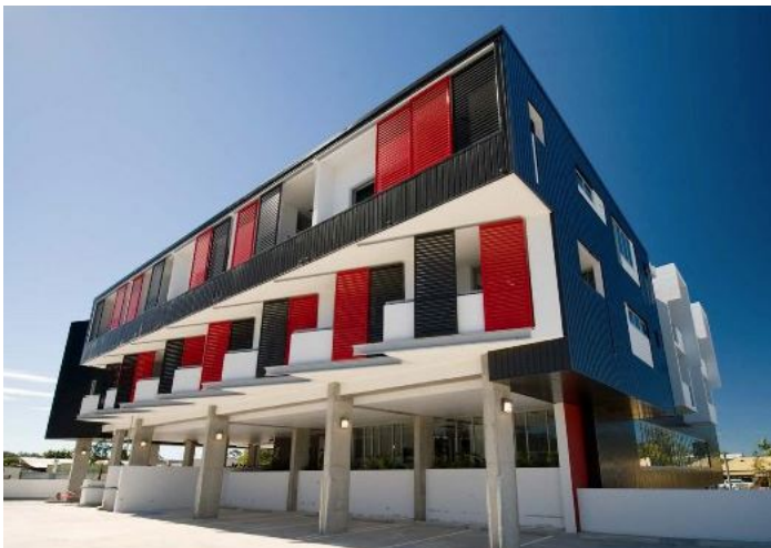
Undercroft parking to the rear of a site not visible from the street.
