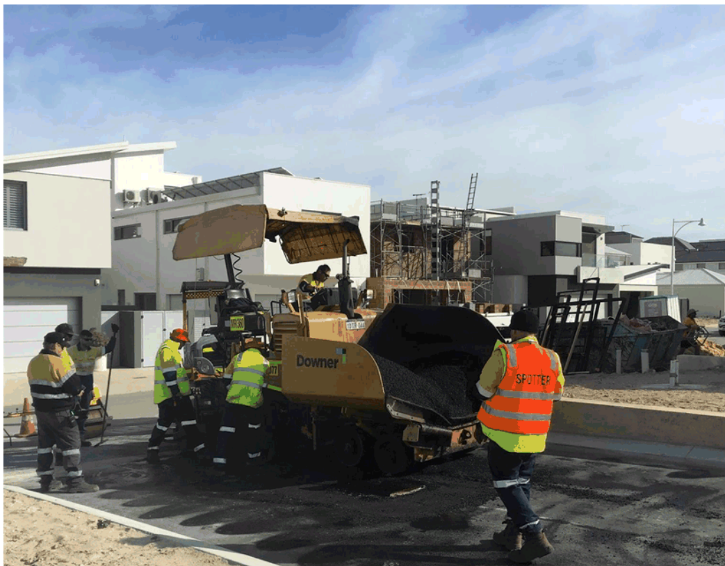
Image 8: A road-surfacing material made from recycled plastic and car tyres (Reconophalt) was trialed on selected roads in Coogee.
