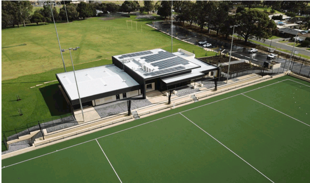
Image 6: The City achieved its renewable energy target. All new community facilities feature solar photovoltaic systems including the Lakelands Hockey and Community Facility (40kW).
