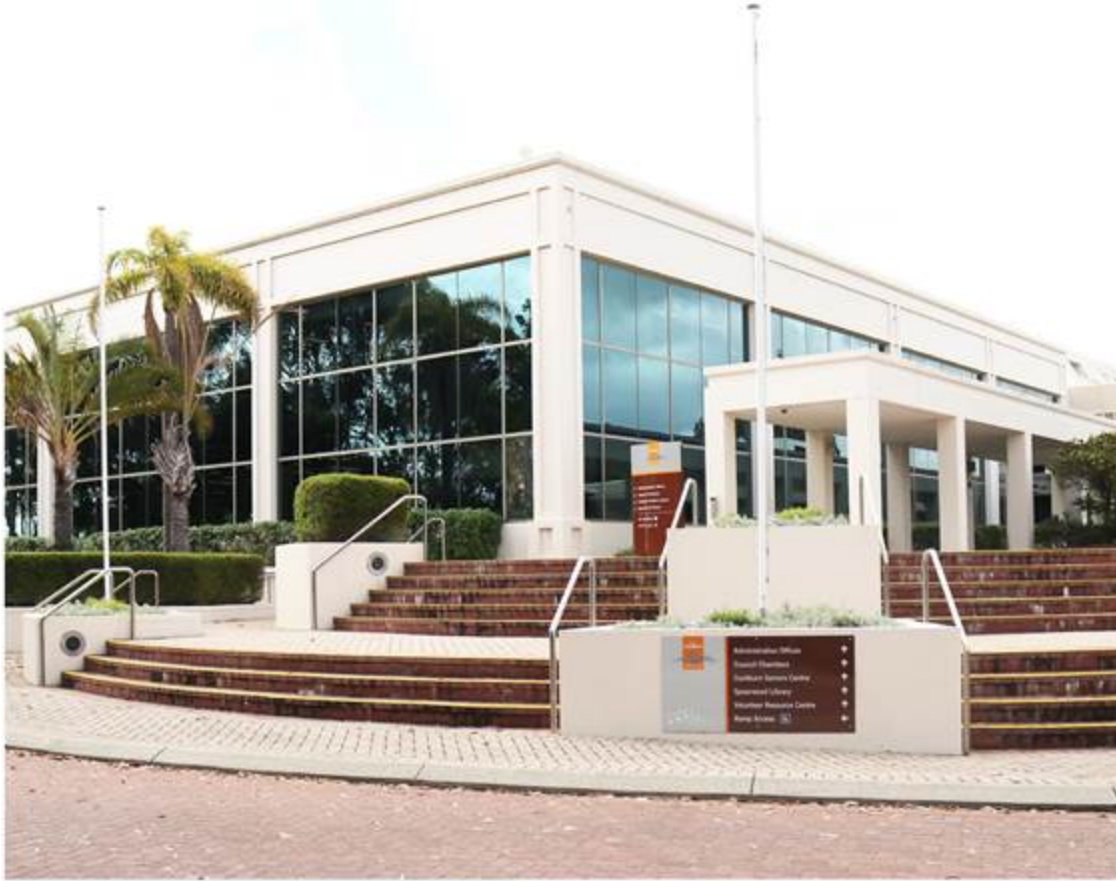
City of Cockburn Administration Building
