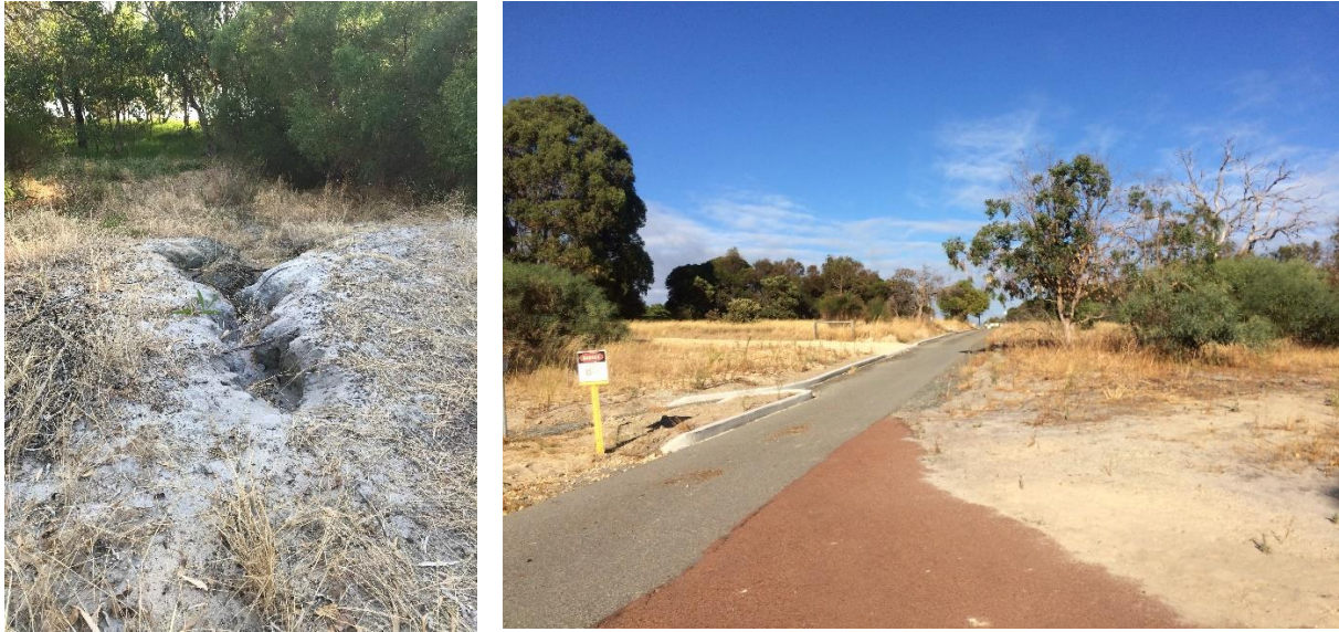
Image 3 Example of erosion caused by stormwater runoff on hard surfaces with mitigation shown on right.
