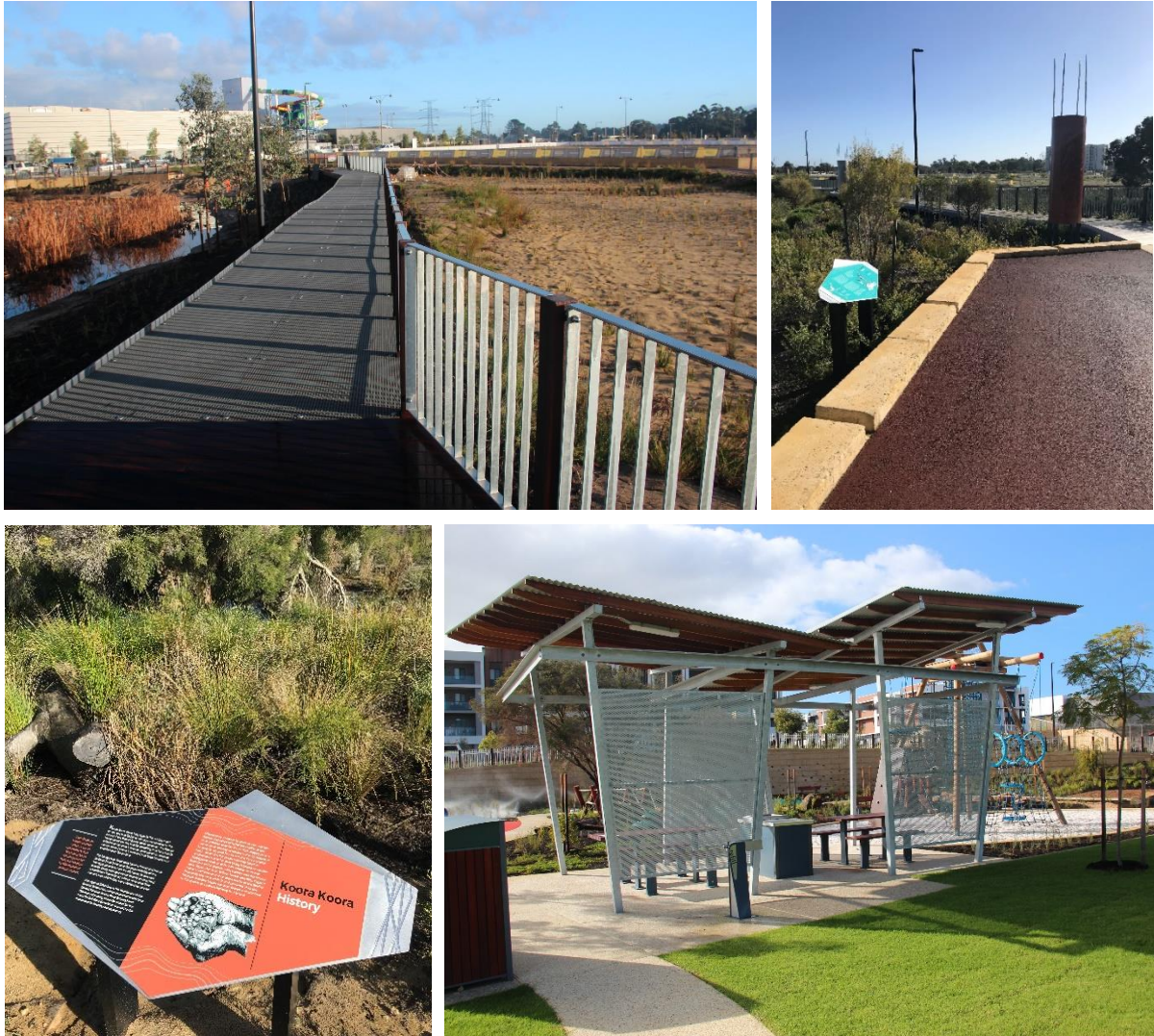
Image 17 Materials and detail of landscape structures that are sympathetic to the natural environment and easy to maintain, examples from Cockburn Central West
