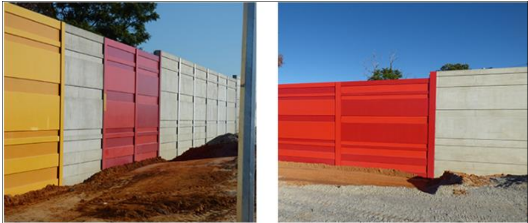
Figure 8 – Examples of Diamond Precast Noise Walls
