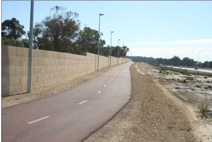
Figure 11 – Examples of Limestone Noise Walls
