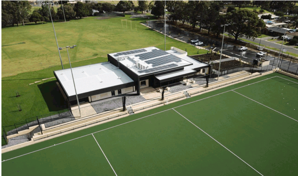
Image 6: The City achieved its renewable energy target. All new community facilities feature solar photovoltaic systems including the Lakelands Hockey and Community Facility (40kW).
