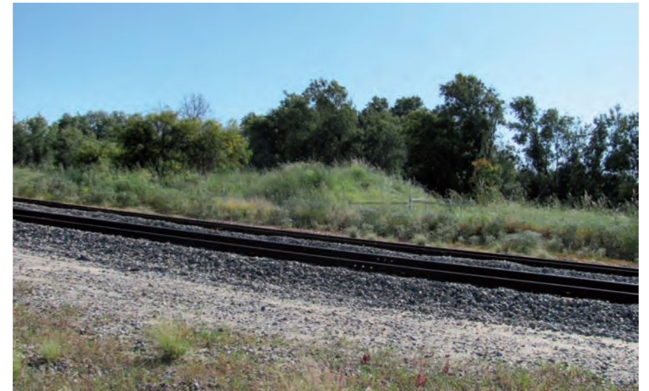
Freight rail infrastructure running through the site
