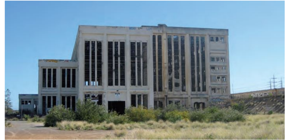
South Fremantle Power Station is a monolithic and historically an important structure
