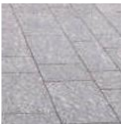
shared path & median_ milled concrete pavers
