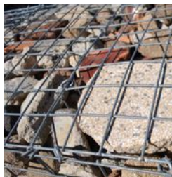
wall material_ gabion walls
