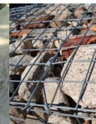
wall material_ gabion walls
