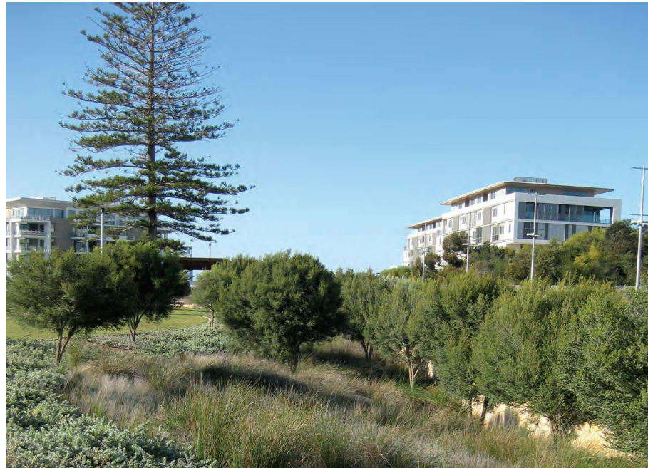
Built form should address green corridors to provide passive surveillance to promote safety
