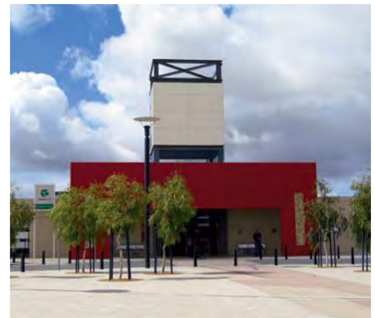
Cockburn Central Railway Station
