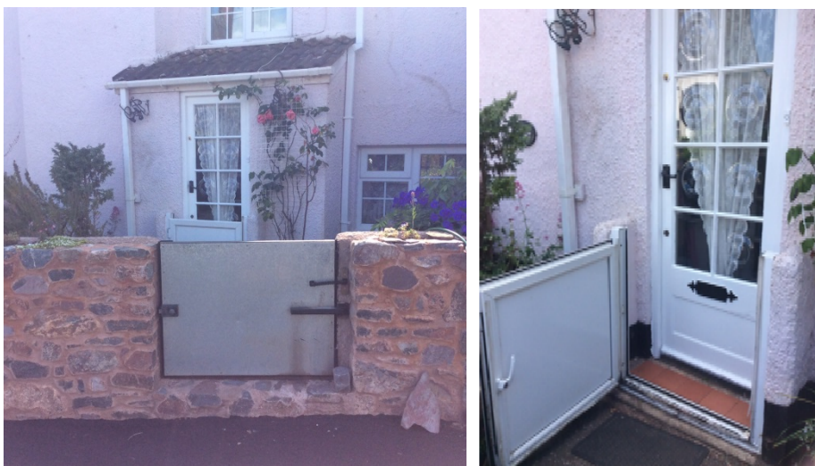
Figure 10 An example of retrospective design requirements: flood wall/gates and doors added to a dwelling to protect existing property from storm related flooding in United Kingdom
