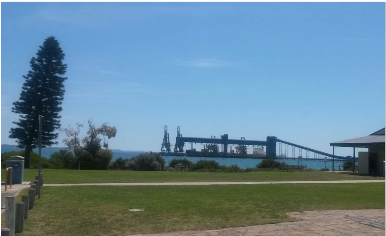
East Rockingham Foreshore showing the grain jetty
