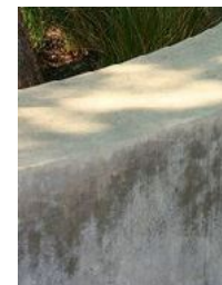
wall material_ formed concrete
