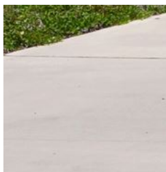
shared path_ brushed concrete
