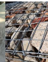
wall material_ gabion walls
