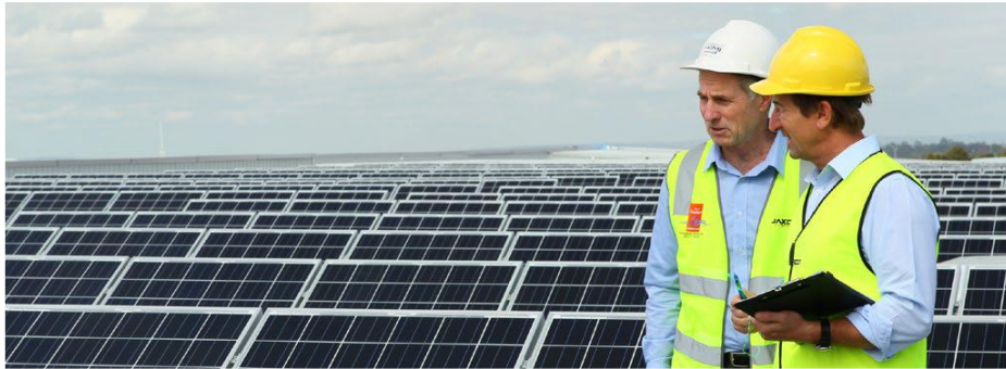
Figure 11: Solar photovoltaic system (130kW), Cockburn Health and Community Facility
