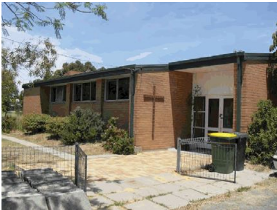
Figure 21: Uniting Church Coolbellup - A small, functional brick church with a brick cross located on the wall near the entrance.
