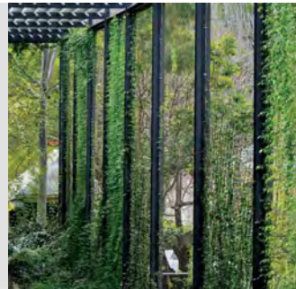
11 RONSTAN TENSILE AGS5 EASY GREENING' VERTICAL CABLE TRELLIS SYSTEM W/ CLIMBING STAR JASMINE TO LANDSCAPE DESIGN SPEC
