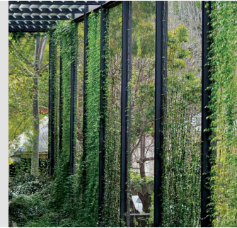
11 RONSTAN TENSILE AGS5 EASY GREENING' VERTICAL CABLE TRELLIS SYSTEM W/ CLIMBING STAR JASMINE TO LANDSCAPE DESIGN SPEC
