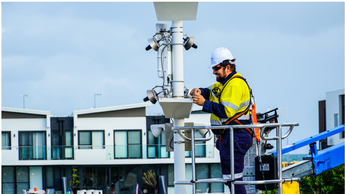
Image 5: LED streetlight upgrade, Port Coogee, June 2020
