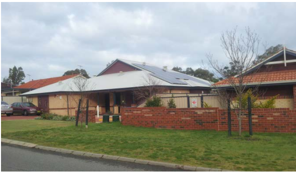
Figure 14. MS Society Care Facility and respite home, Hamilton Hill
