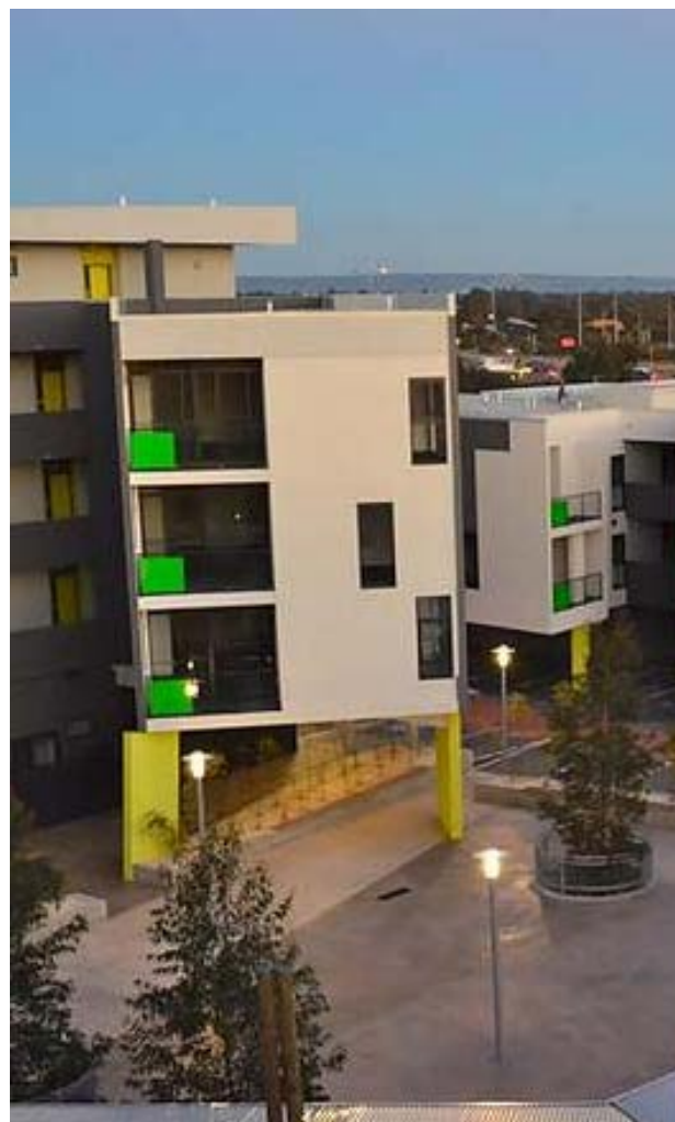
Figure 1. Apartments in Cockburn Central – A transit oriented development.
