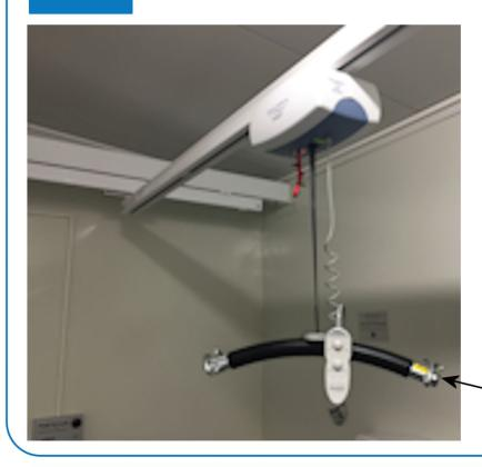
Hold and use the spreader bar to pull the hoist into a clear area for safe use. Make sure there are no obstructions around you
