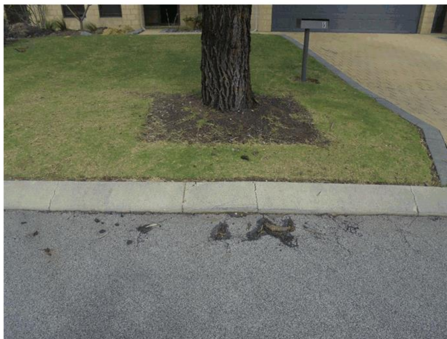
Figure 3 Displaying surface roots emerging from the asphalt roadway and associated damage.
