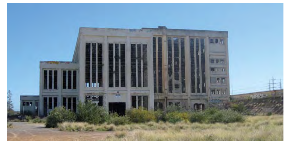
South Fremantle Power Station is a monolithic and historically an important structure
