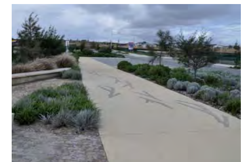
Broom finished concrete paths
