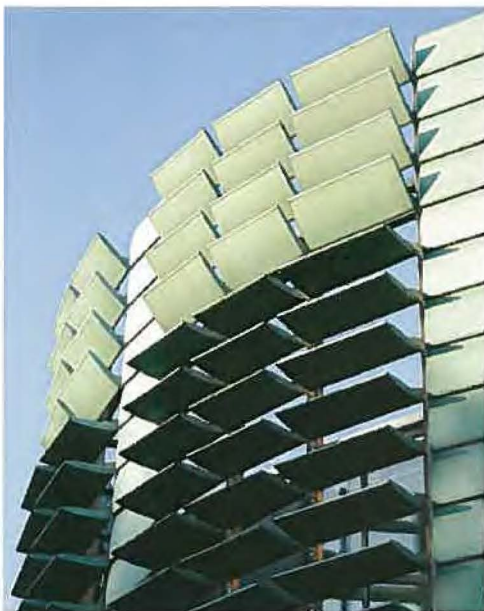
HORIZONTAL LOUVERS OFFER PROTECTION TO WINDOWS
