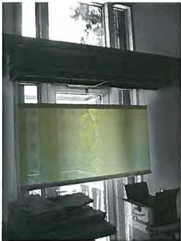
SUSTAINABLE DESIGN-BLINDS THIS BLIND HAS BEEN SHORTENED AND IS MOVED ACCORDINGLY TO PROVIDE PROTECTION FROM DIRECT LIGHT AND ENSURE AMBIENT LIGHT ENTERS THE OFFICE SPACE, THEREBY REDUCING RELIANCE ON ARTIFICIAL LIGHTING.
